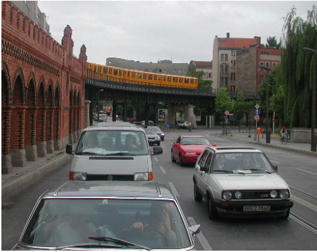
30. The plan recognises the need for an integrated land use and transportation system, which has the potential to cater for different modes.
